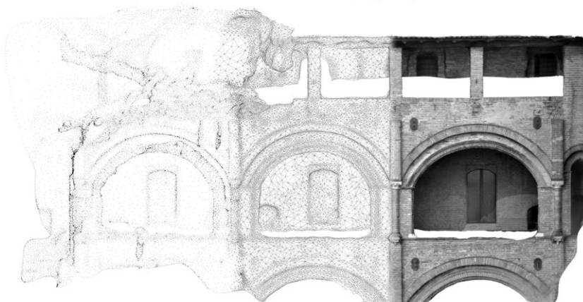
Fig. 2. Three-dimensional "collapse digital model" of the Finale Emilia Castle Fortresses loggia obtained with automatic development process (image matching) using the software 123D Catch by Autodesk by the students of the course: Maria Giovanna Rizzi, Serena Schiraldi, Gaia Spagnoletti, Graziana Tagarelli, Federica Vitarelli e Valentina Zaza.
