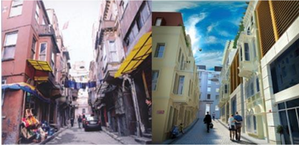
Fig. 13. Tarlabası Urban Renewal Project, original urban fabric and new project site-4.
