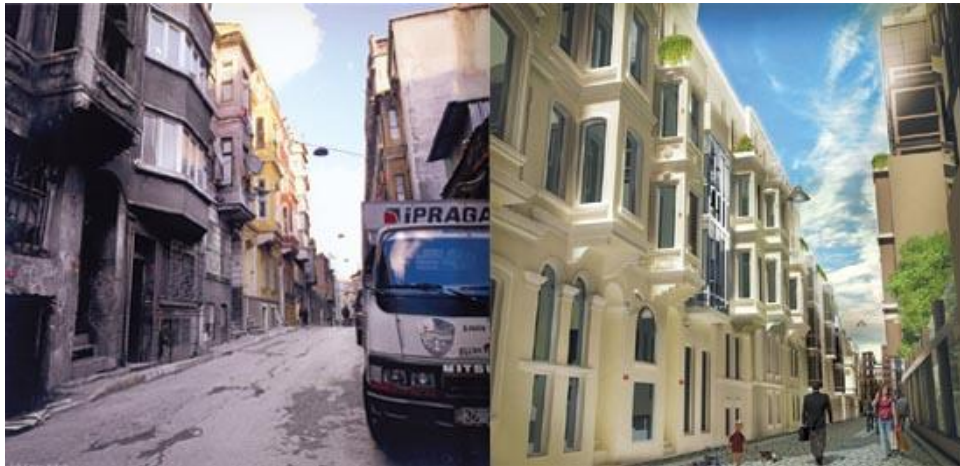
Fig. 14. Tarlabası Urban Renewal Project, original urban fabric and new project site-5.
