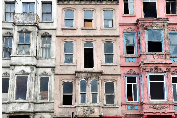
Fig. 1. An example of the row houses in Tarlabası. (Before demolition)
